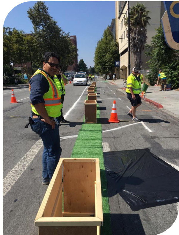
City of San Jose staff and volunteers install a temporary pop-up cycle track on Fourth Street to demonstrate the city's plans for a connected network of protected bikeways in downtown. The reusable, portable planter boxes were borrowed from Mountain View's local bicycle advocacy group, which loans them out for demonstrations like this one. Photo: Jessica Zenk
