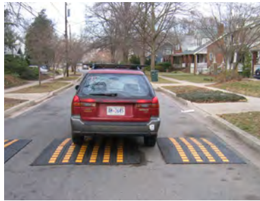
Vertical deflection: includes raised crosswalks, speed cushions, and speed humps
