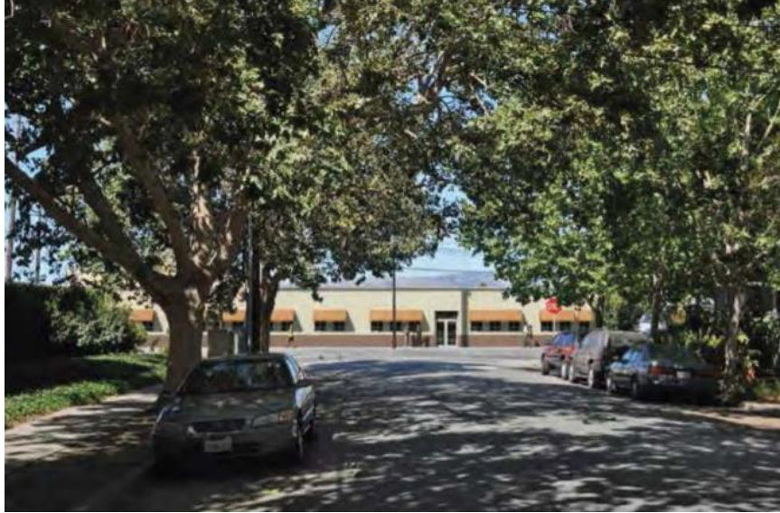
Example of a mid-tunnel facility on Stockton Avenue Source: Final SEIS/SEIR
